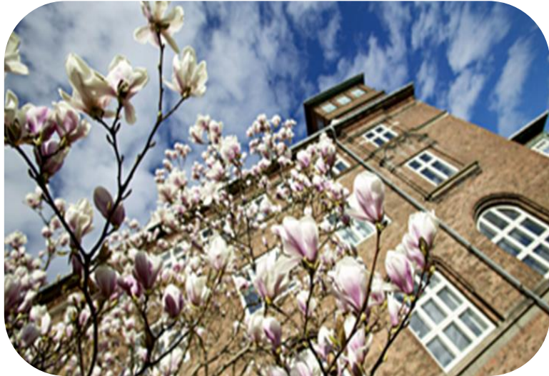
Case 1, Denmark Bispebjerg Hospital (BH) 2010-2012
